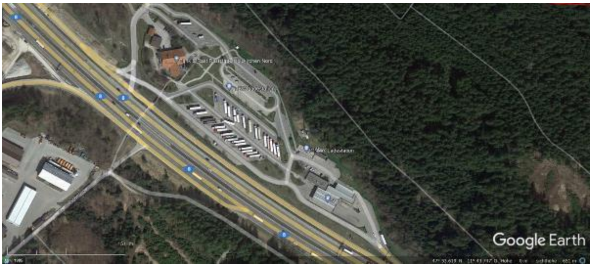
Figure 17: Example for a big parking site with extended infrastructure
