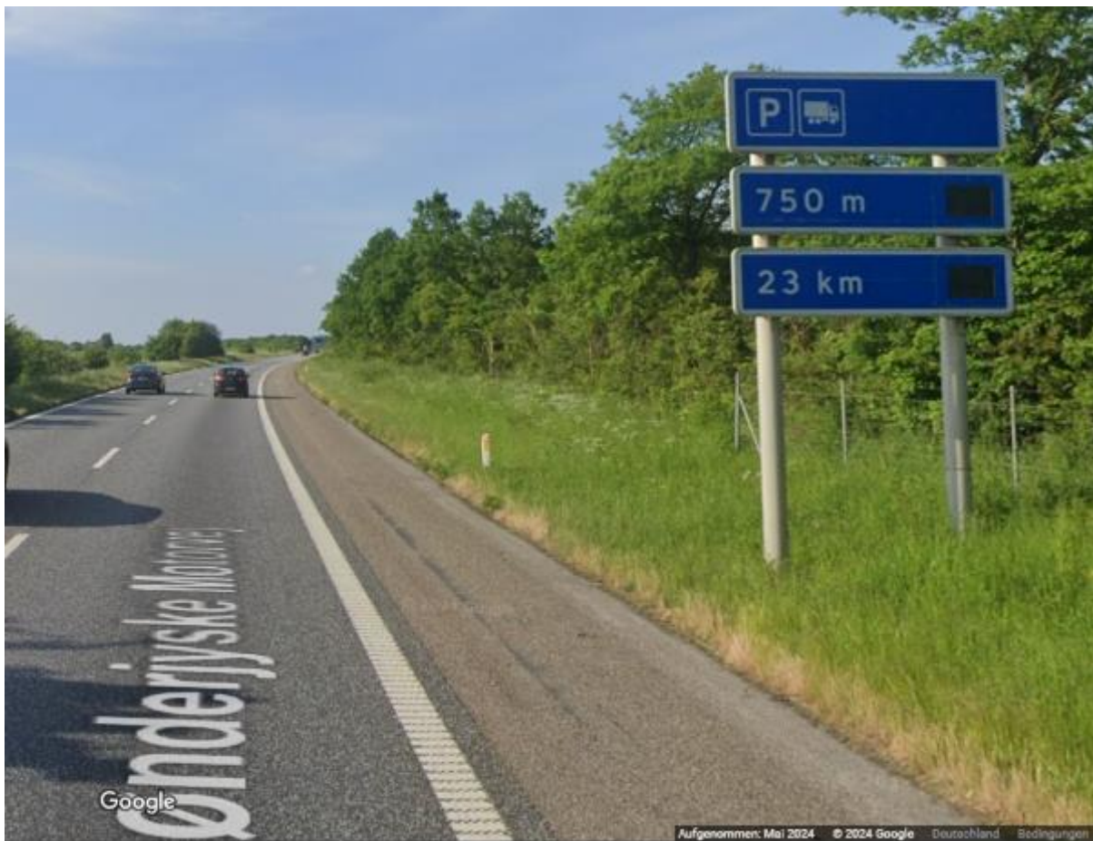
Figure 14: Example for parking site at the E45 with a classical arrangement of parking places in one row.
