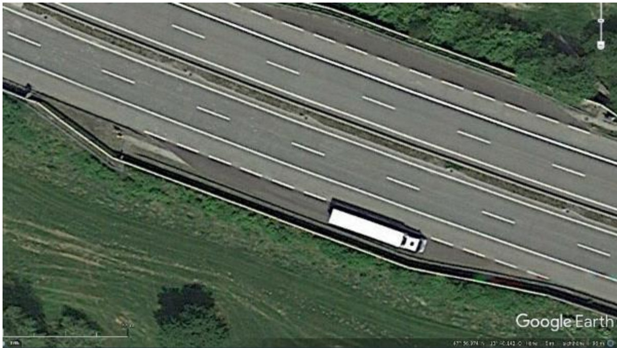
Figure 1: Example for a parking truck in an emergency lay-by
